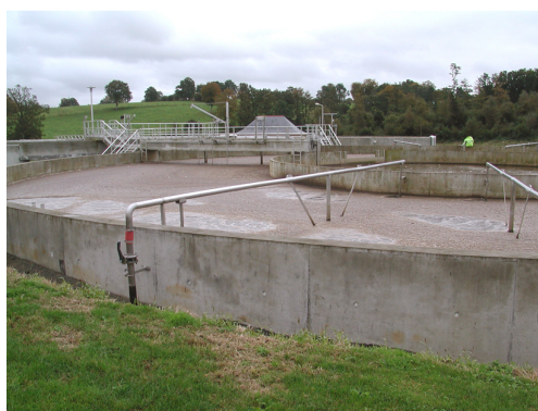
"Illustration 10" Station d'épuration PAP/CRCK du Centre
